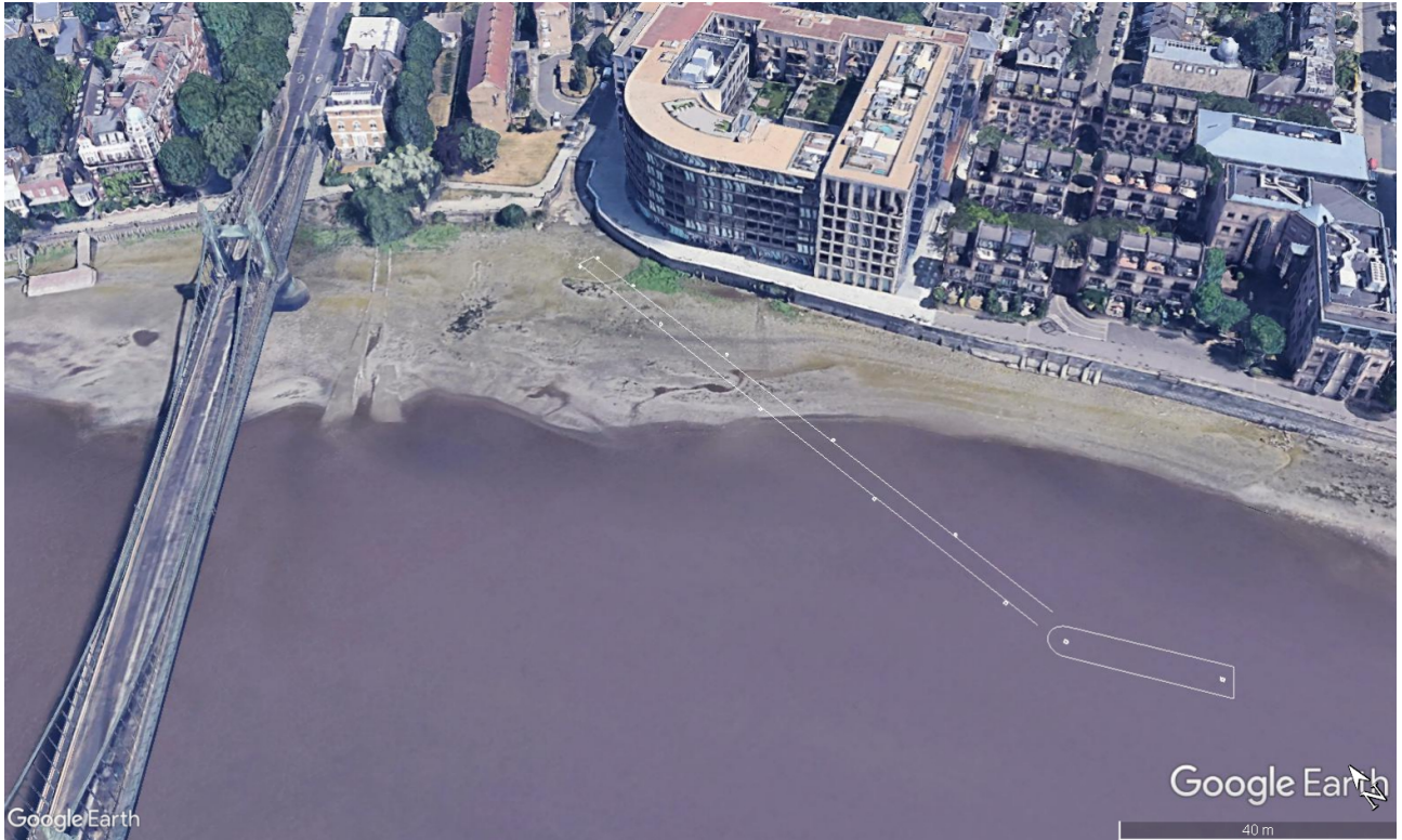
Figure 4.12: Drainage channels evident on the foreshore beneath the floating walkway
