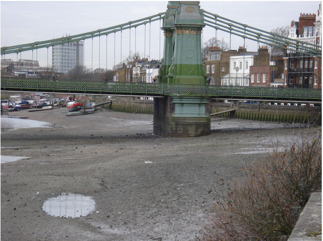
Photograph 3.1: Hammersmith foreshore: sand and gravel foreshore composition
