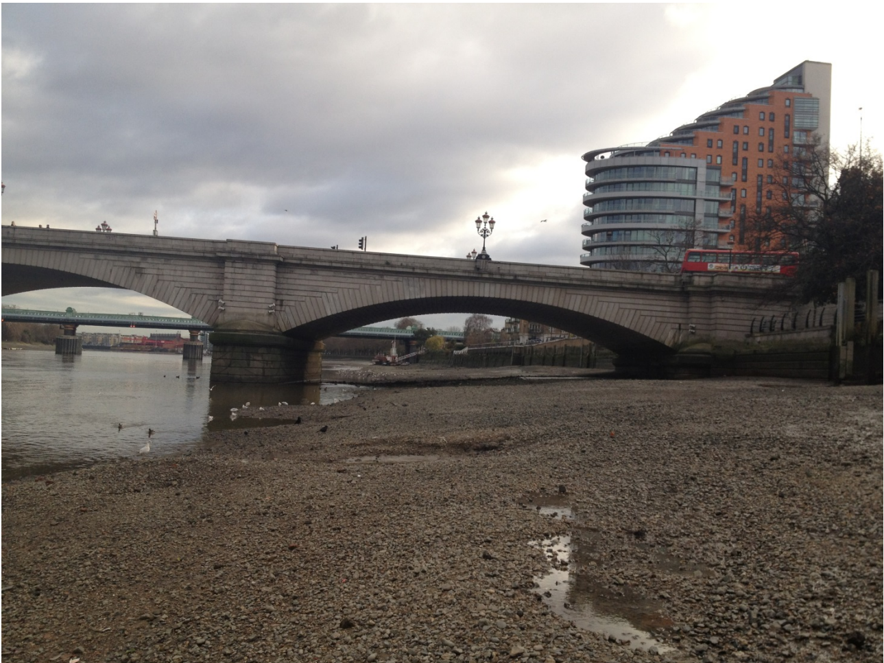
Photograph 4.1: South foreshore at Putney Bridge
